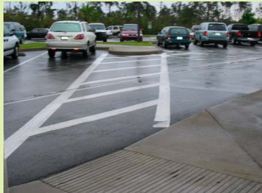
A crosswalk connects a curb ramp to a sidewalk without a curb ramp
